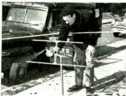
Edward Weigand, Farr service man, sprays Krylon on entire antenna. Krylon shuts out moisture, rain, salt spray—prevents corrosion and pitting—keeps picture quality at peak.
